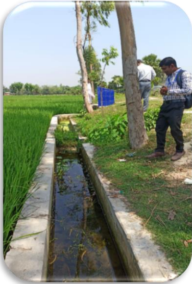
Image 3.2: Inspection of Irrigation Drain, Mahadevpur Upazila, Naogaon
