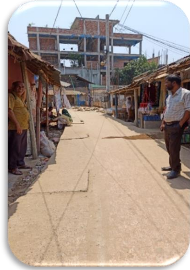
Image 3.4: Road Inspection, Sapahar Upazila, Naogaon
