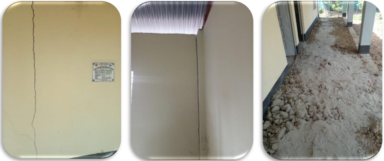
Image 3.6: Nandigram Technical and Business Management College, New Building Construction Project, Nandigram Upazila, Bogra
